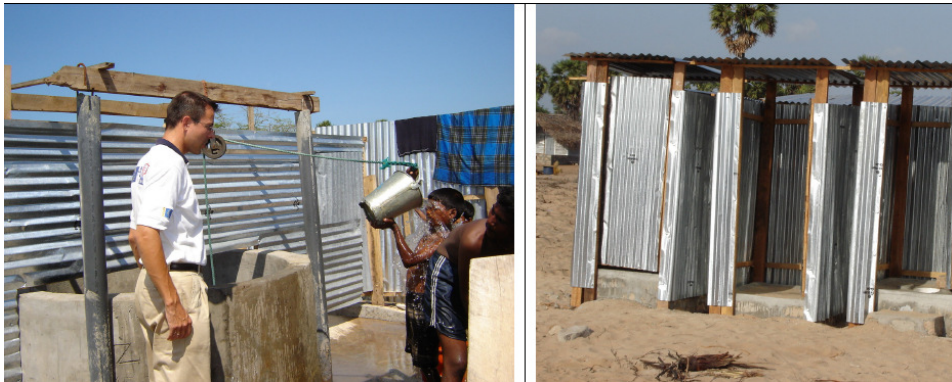
Figure 5: Semi-permanent watsan facilities in Tsunami transitional camp
