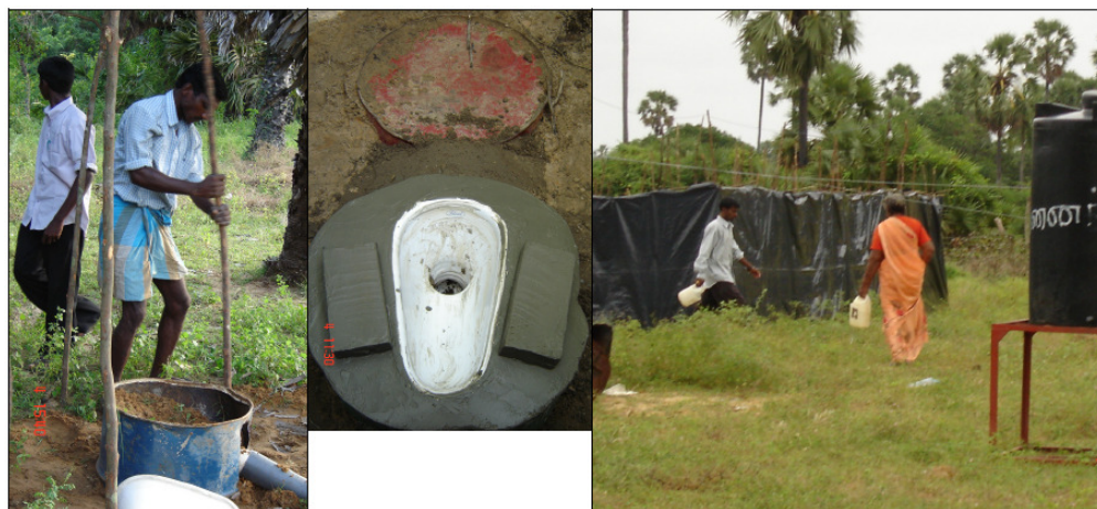
Figure 2: Constructing temporary toilets with local materials
