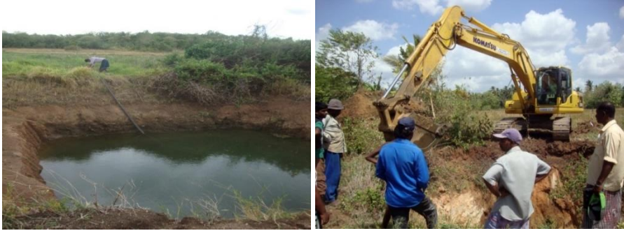
Figure 3. An improved existing well and construction of a new well
